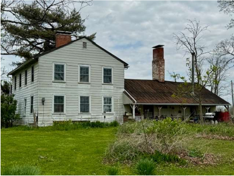
Figure 2 Rear of the single-story and two-story structures which formed a single building.
