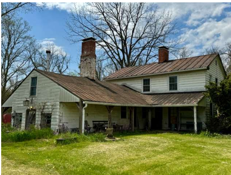
Figure 1 The single-story structure is the original Potter's tavern building. Both structures were built in the early 1800's.
