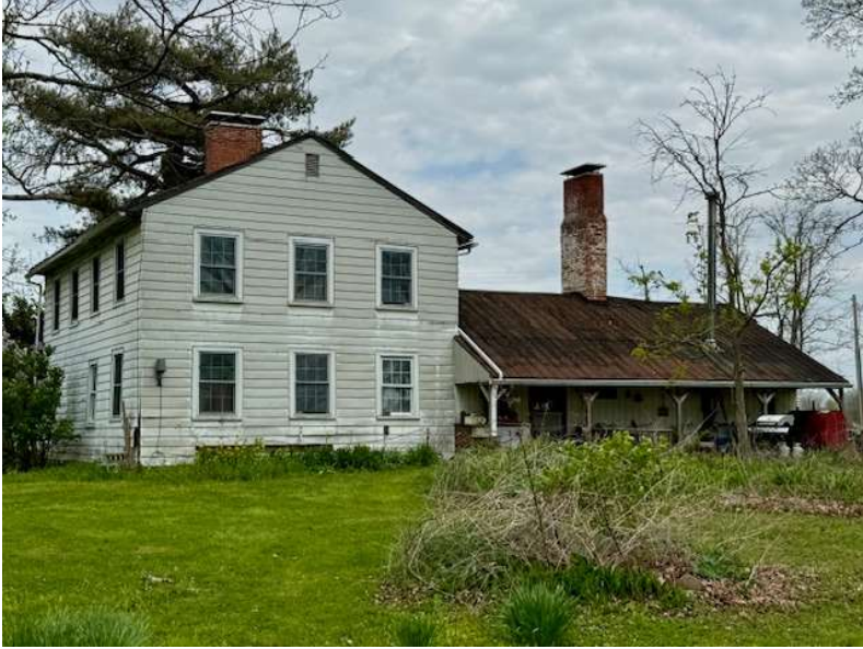
Figure 2 Rear of the single-story and two-story buildings.
